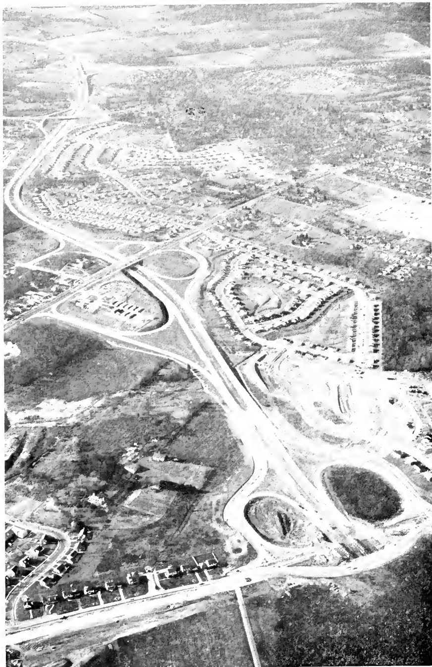
Baltimore Beltway, showing interchanges at the Baltimore-Harrisburg Expressway, the extension of Charles Street, York Road, and Dulancy Valley Road. The Beltway is now extended east of the Dulancy Valley Road.
